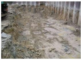
Muddy site conditions due to the presence of seawater below ground, led to difficulties on-site
