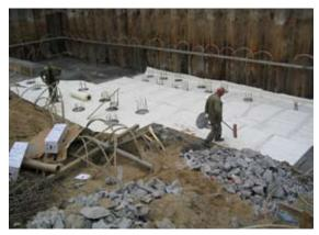
Preprufe being installed below the slab
